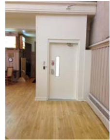
Completed 2 nd lift
