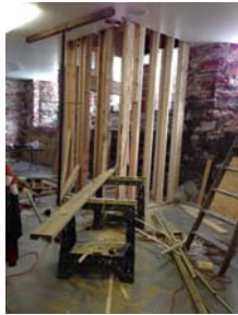
Prep work downstairs
