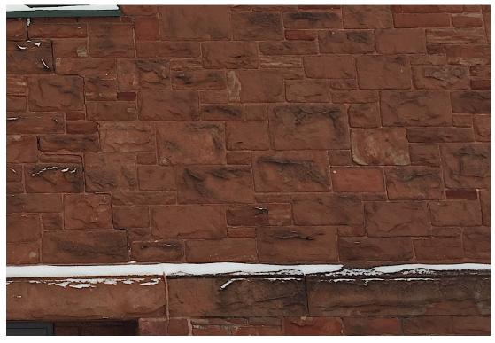
Mortar between the sandstone block deteriorates, causing the blocks to shift and leak. Both the back and front of the building had places with significant deterioration. A few places on the sides showed problems and repairs in the stones around the glass blocks were needed.
