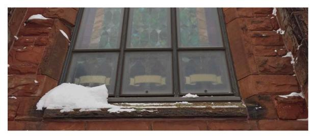
Stained glass windows were restored, repaired or replaced in 1997. 20 years of weather have taken their toll on some of the frames.
