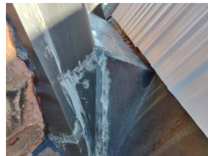
Patching, plugging, and pointing
